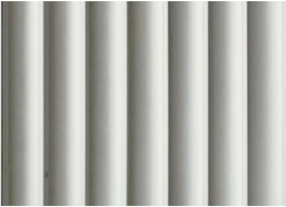
401 LOUVRES SCREEN 01 TYPE 1 COLOUR: POWDERCOAT SURFMIST
