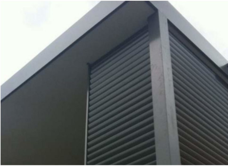
403 LOUVRES SCREEN 03 TYPE 3 COLOUR: POWDERCOAT MONUMENT
